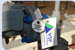
Screen Gasket installed in flange
