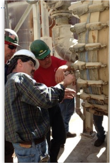
VSP Engineer Providing On-Site Field Support
